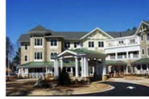
Senior Living Facility
